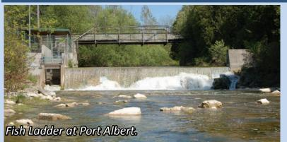
The Port Albert Fishway (PAF) was constructed at the historical mill dam in the village of Port Albert, to allow the passage of spawning fish to upstream coldwater streams in the Nine Mile River Watershed.
